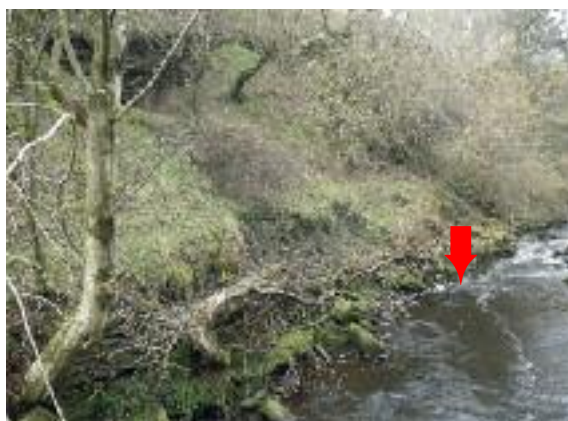
Fig 3.1.2 Living tree is laid to reduce river bank collapse at old quarry / mine site. Additional trunk is secured on the river bed to direct flow away from eroding bank. One season of growth demonstrates how well the bank is repairing. This is a fixed point photography site (from marked post on footbridge).
