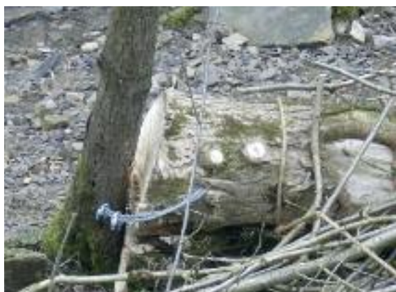
Fig 3.1.3 Usual hemp rope which will degrade in time as the trunk / brash bed into position is augmented by 6mm tensile cable threaded through live growing tree and felled trunk to ensure trunk does not detach in high flows and cause damage downstream.
