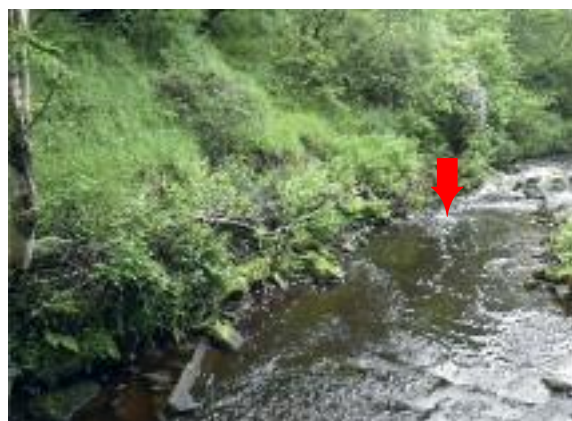
Fig 3.1.2 Living tree is laid to reduce river bank collapse at old quarry / mine site. Additional trunk is secured on the river bed to direct flow away from eroding bank. One season of growth demonstrates how well the bank is repairing. This is a fixed point photography site (from marked post on footbridge).
