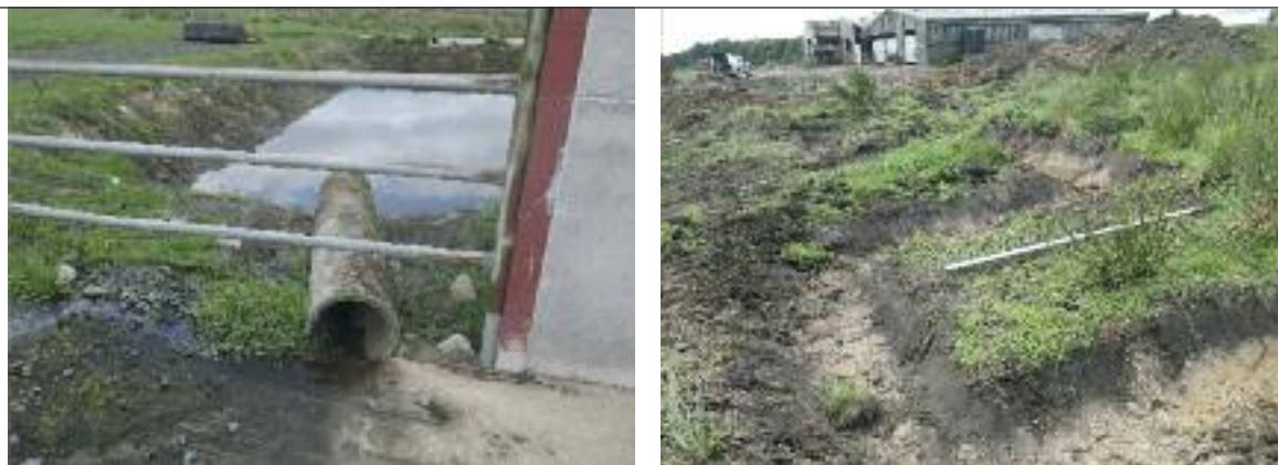
Figure 3.2.1 First settlement pond, also showing access track for emptying the pond, reinforced wall and stock proof fencing (left). Winding settlement channel with first settlement pond, farm buildings with guttering and water tanks in the back ground (right).
